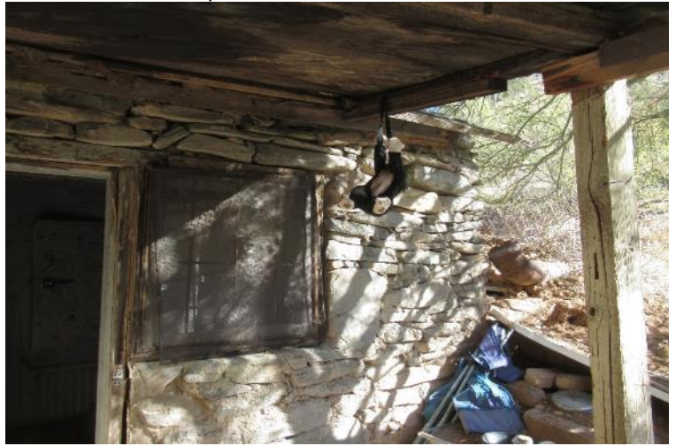
Within about an hour and half, they arrived at the mine site and came across this cabin.
